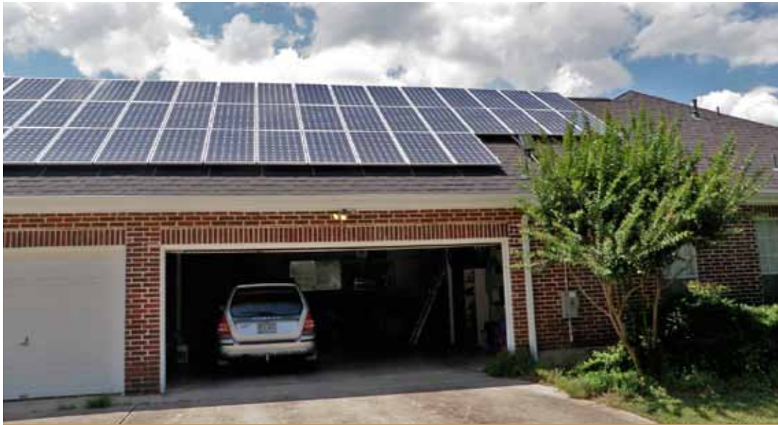
A solar energy system installed on the roof of a house in San Antonio with the help of CPS Energy.
